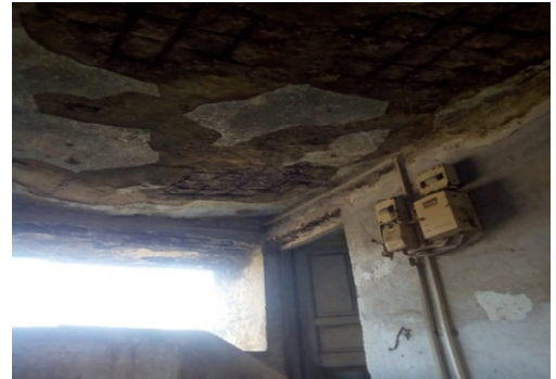
Police hospital running in extremely damaged building at JAP 6 battalion at Jamshedpur (28/11/2018).
