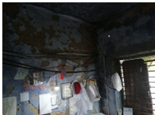
Poor condition of building of Meharma PS, Godda (10/10/2018).
