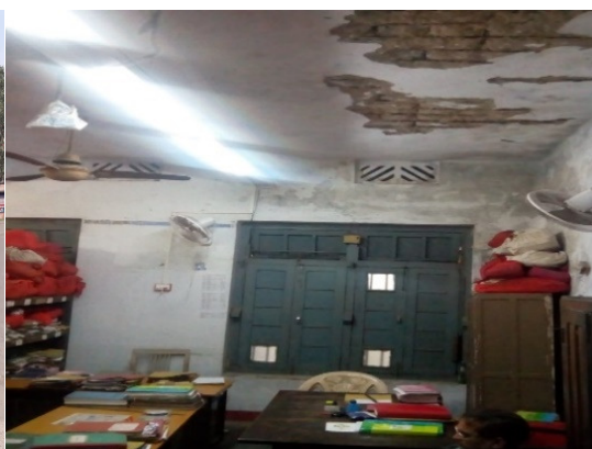
Room with damaged ceiling being used as Reserve Office at East Singhbhum PL (23/10/2018).
