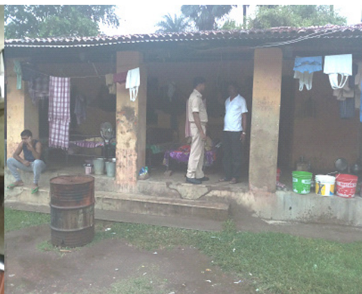
Dilapidated verandah of PL used as barrack by police personnel of Godda district (12/10/2018).
