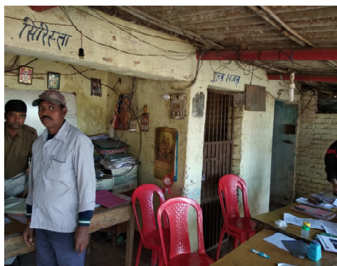
Congested and poor condition of building of Nagari PS, Ranchi (20/12/2018).
