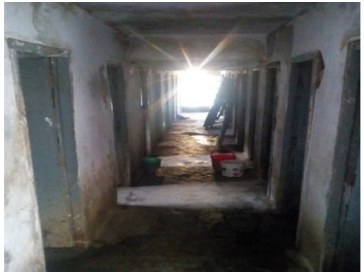
Poor condition of toilets inside barrack of JAP 6 at Jamshedpur (28/11/2018).
