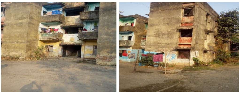
Condemned residential quarters at JAP 6, Jamshedpur still in use (28 November 2018)
